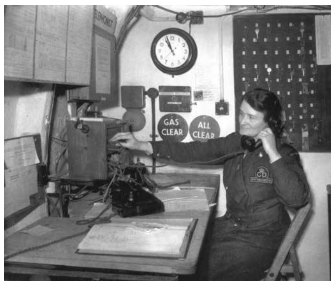
The shelter warden in the control room
